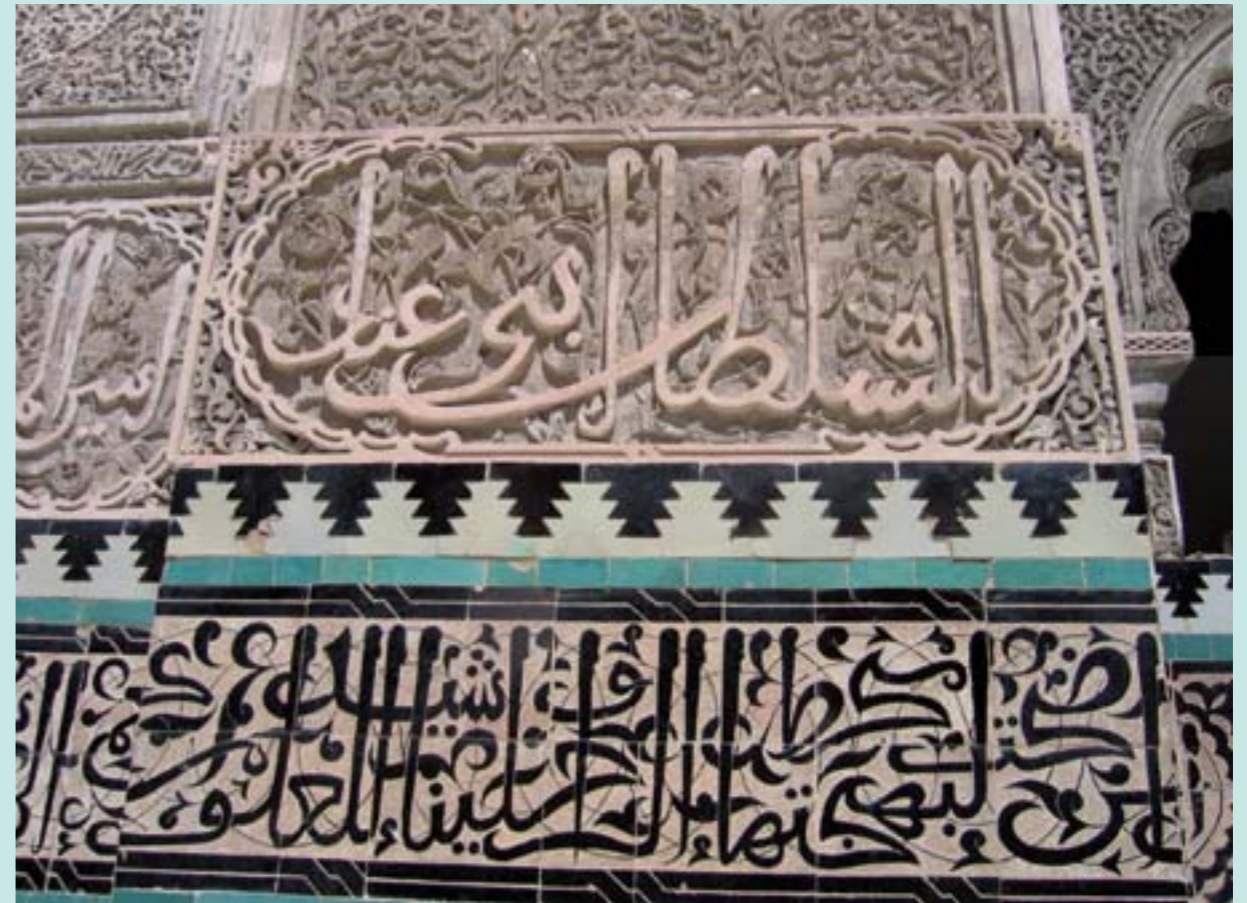
The extraordinary delicacy of Fassi craftsmen's work is fully apparent in the zellij and carved stucco work they create
